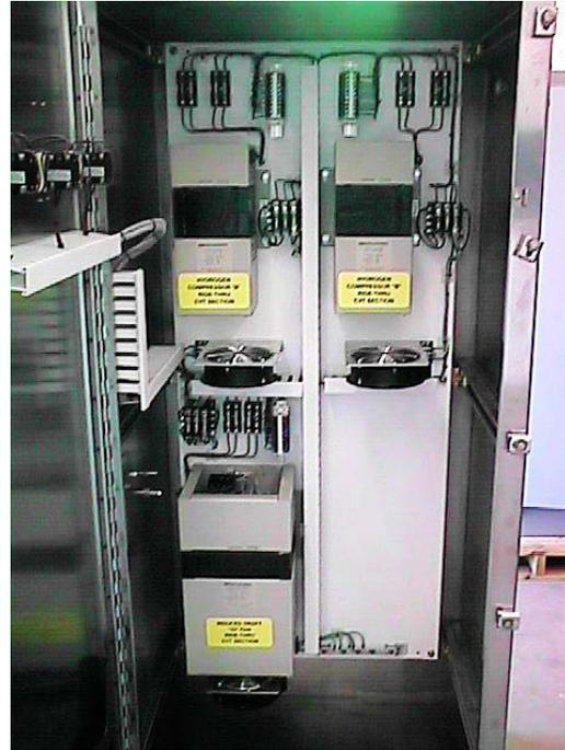
Figure 6. CVT enclosure internal components i.e. CVTs, fans, fuses, and termination blocks.
